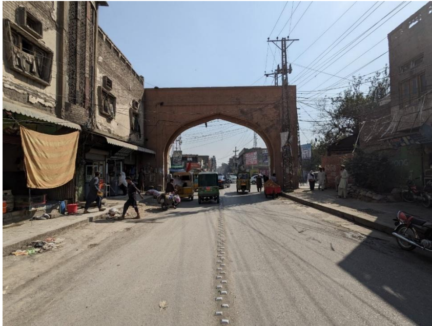
Figure 12: Clock Tower Area
